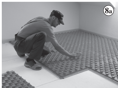
Insulation panel laying
