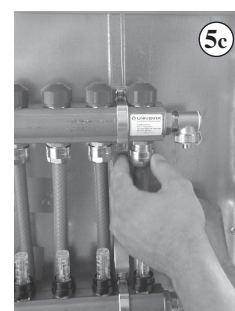
Pipe attachment to the manifold
