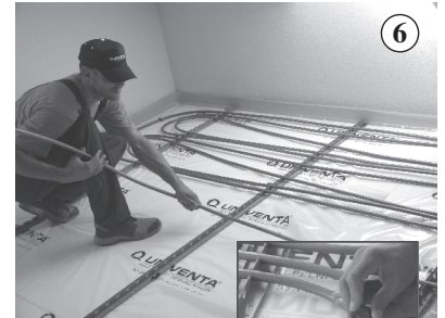
Heat pipe laying
