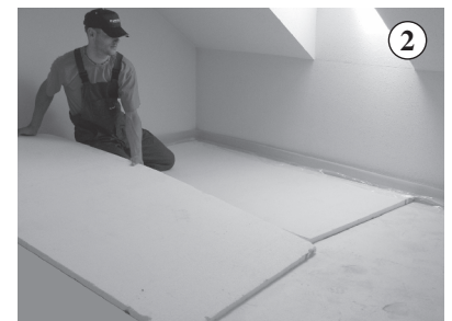
Thermal insulation laying
