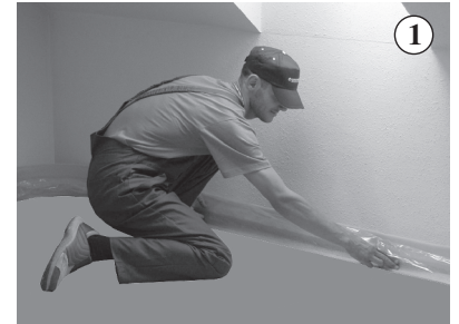
Expansion strip laying
