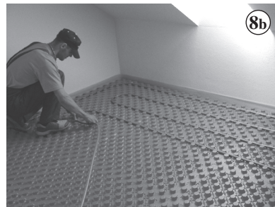
Heat pipe laying
